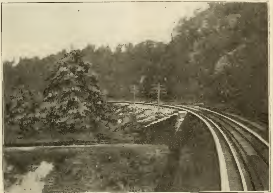
VIEW TAKEN FROM THE CAB WINDOW OF A MOVING ENGINE. THE NARROWS, ABLEMAN'S, WIS.
